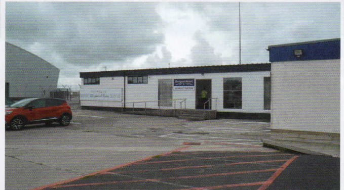
The old terminal building has been replaced by this
